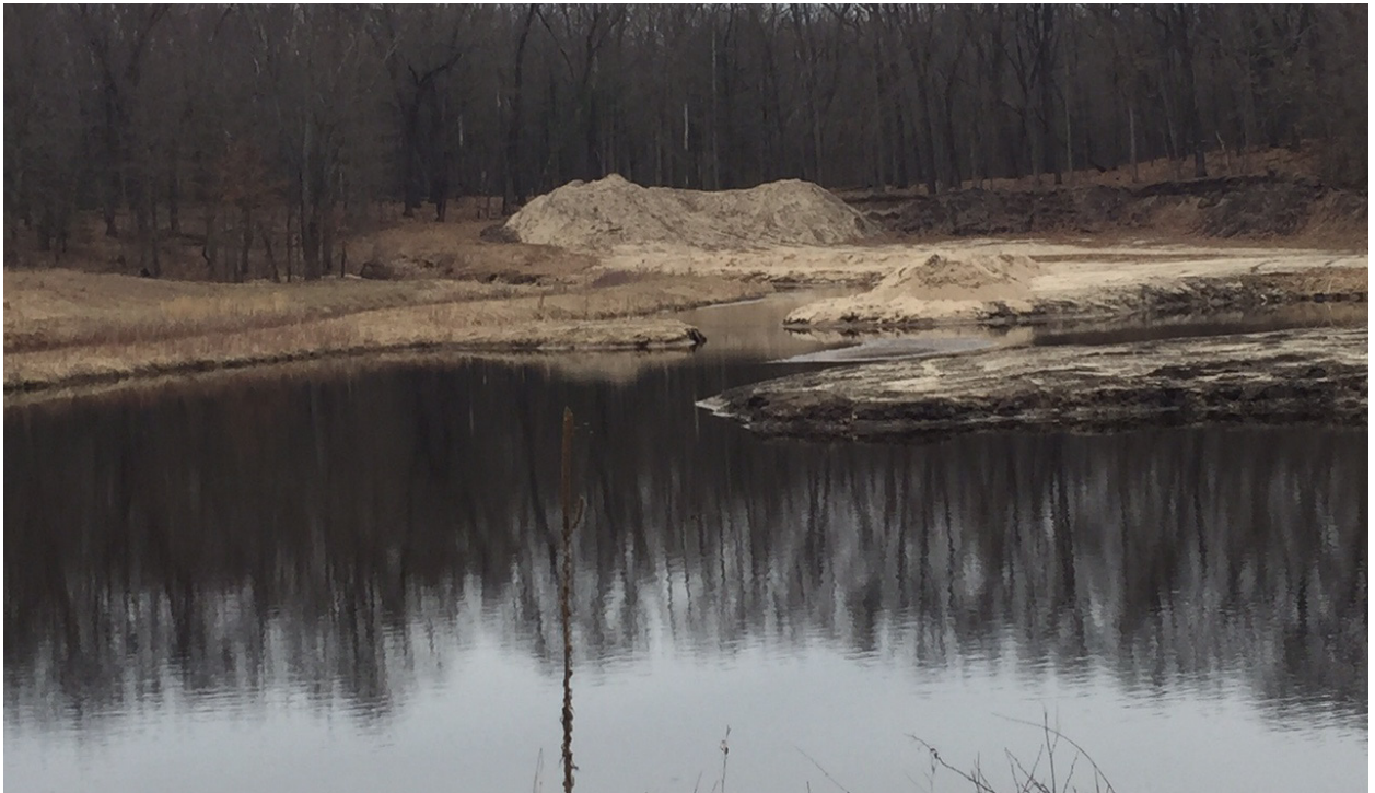
Figure 23. Wheeler Drain sediment basin south of Hess Lake Drive.
